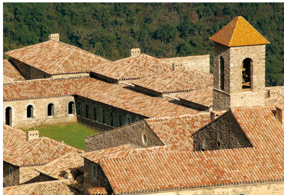
Renovation of Notre-Dame de Clémence Monastery at La Verne >
